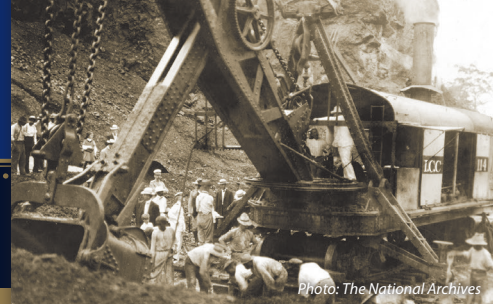
President Theodore Roosevelt controls a steam shovel while inspecting Panama Canal construction, November 1906.
