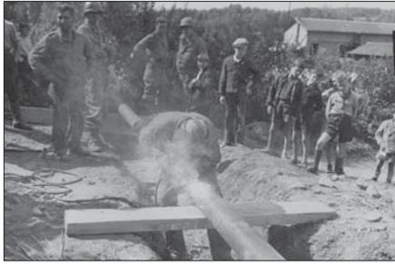
Engineers weld a gasoline pipeline into place to meet the demand for fuel by the advancing Allied forces.
