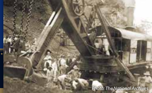
President Theodore Roosevelt controls a steam shovel while inspecting Panama Canal construction, November 1906.
