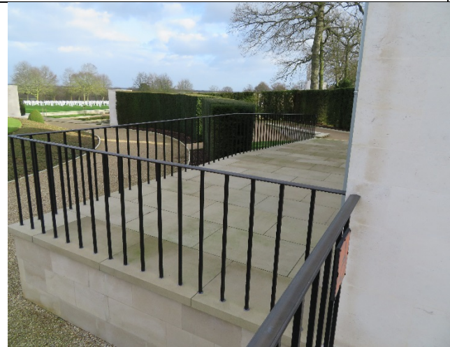
Ramp from entrance courtyard to lower level
