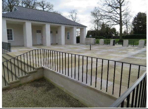
Level entrance courtyard and accessible toilet
